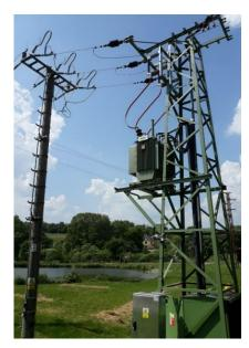
CEZ Distribuce installed Voltage regulated distribution transformers from SGB Company equipped with Maschinenfabrik Reinhausen On Load Tap Changer (OLTC) in 3 demonstration areas, in order to enhance testing. OLTC enables to test the behaviour of the autonomous functions at any time without waiting for voltage change in the grid.
