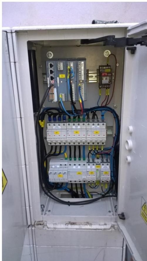
Figure 43- LV cabinet with ripple control receiver and RTU in Decin
