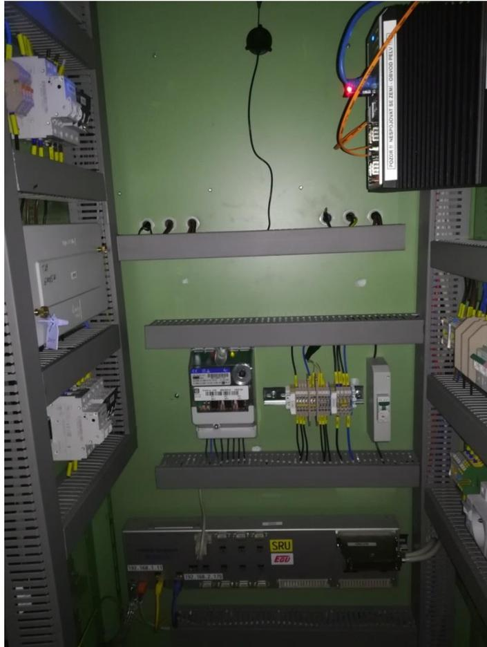
Figure 27 - CEZ Obnovitelne zdroje - local control system SRU (slave) used for volt-var control at small hydro Vydra 6.4 MW
