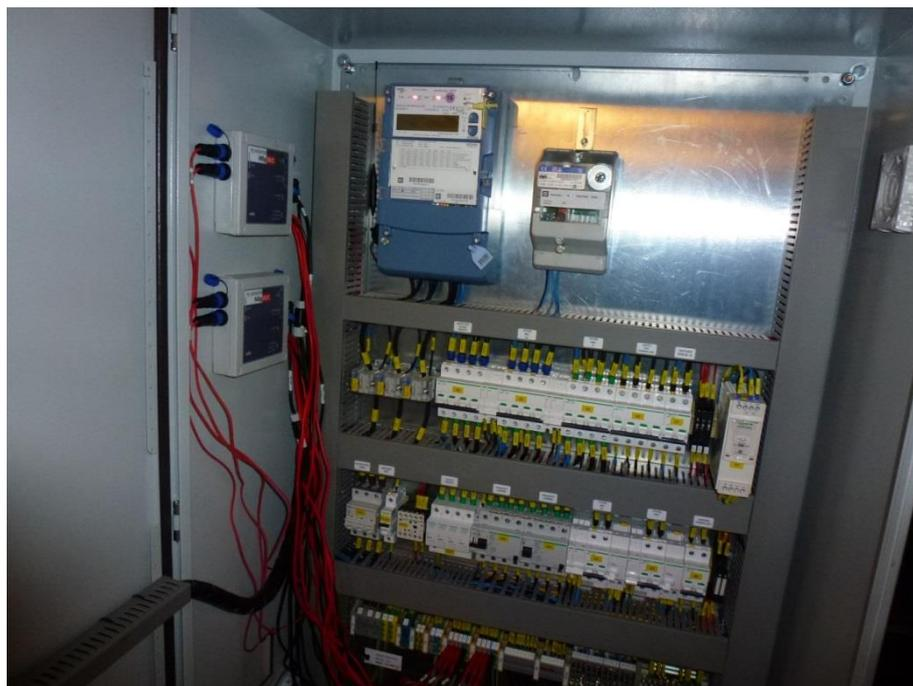
Figure 41- LV cabinet with billing meter, ripple control receiver, RTU and two MEg38 power quality measurement devices in Hradec Kralove
