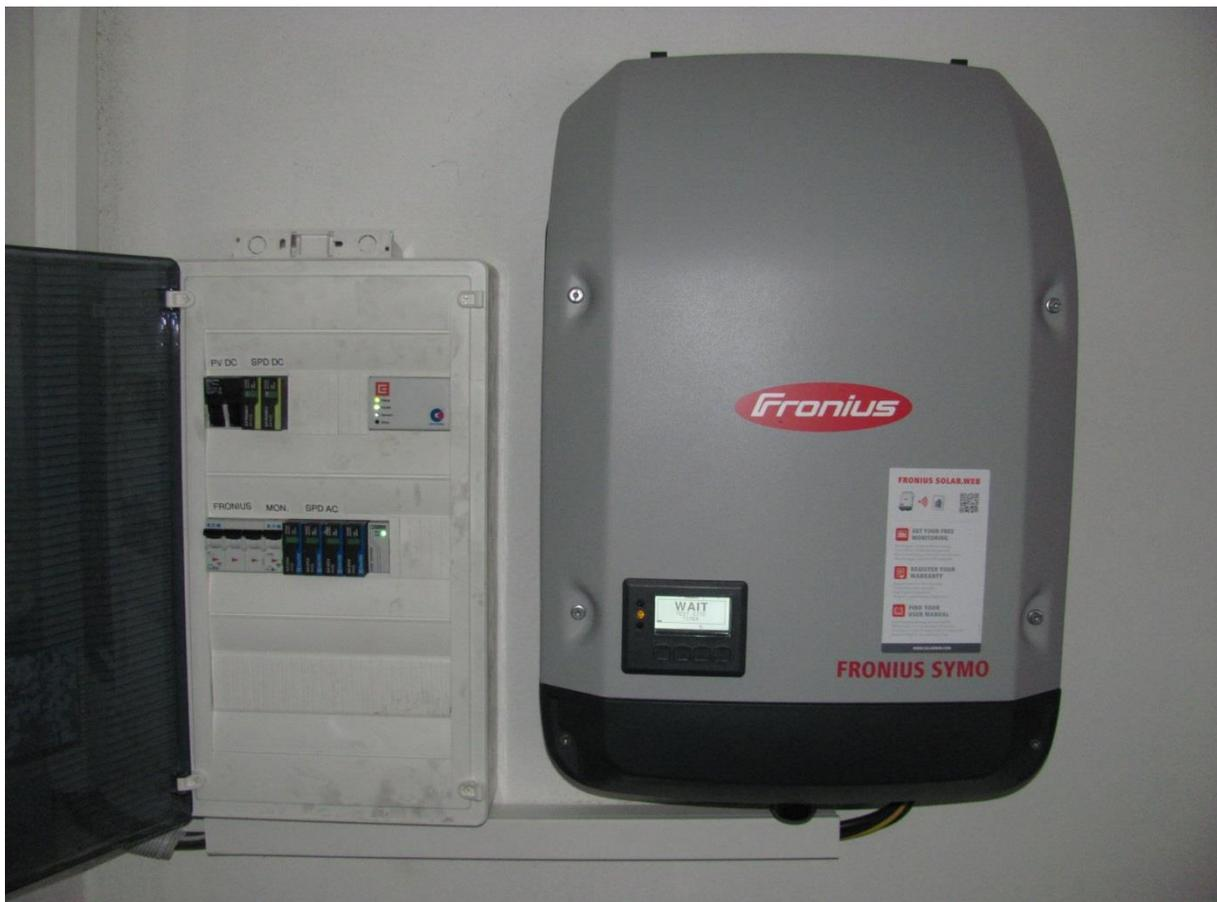
*Figure 14 - Fronius Symo smart PV inverter installed in Divisov area (the same type of PV inverters is used on all PV installation in Divisov and Teptin areas which are included in the InterFlex project)*
