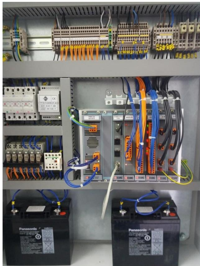
Figure 31 - PV Zamberk 1.1 MWp - LV cabinet with RTU which has GPRS/LTE connection towards CEZ Distribuce SCADA and which includes volt-var control algorithm
