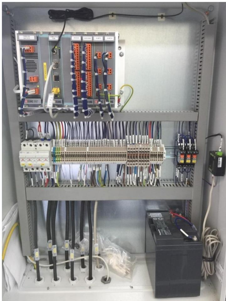
Figure 34 - wind park Koprivna 4.6 MW - LV cabinet with RTU which has GPRS/LTE connection towards CEZ Distribuce SCADA and RS485 connection with control system which secures volt-var control at targeted voltage set point
