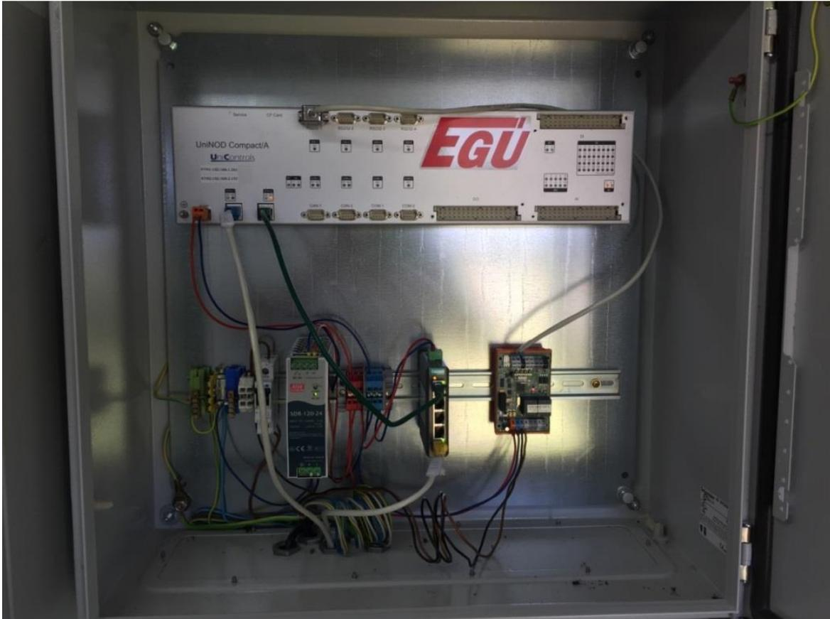
Figure 35 - wind park Koprivna 4.6 MW - LV cabinet with control system which control reactive power of wind park generators and which secures volt-var control at targeted voltage set point
