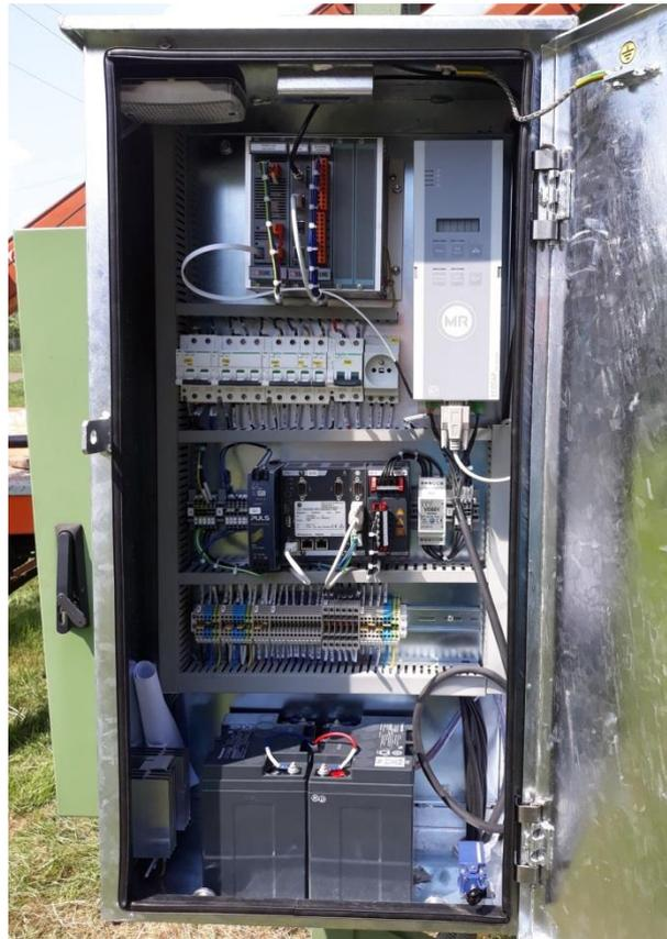
Figure 17 - LV cabinet with RTU and OLTC regulator installed in Divisov area
