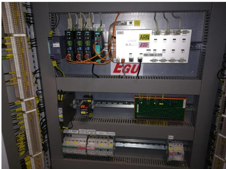
Figure 26 - CEZ Distribuce - local control system ARN (master) used for sending commands towards volt-var control system (SRU) at small hydro Vydra 6.4 MW
