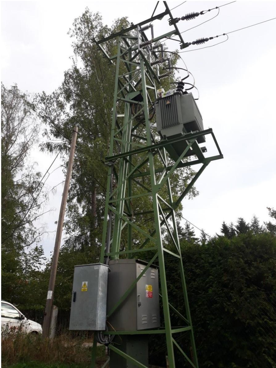
*Figure 16 - Voltage regulated distribution transformer 22/0.4 kV with OLTC installed in Teptin area*
