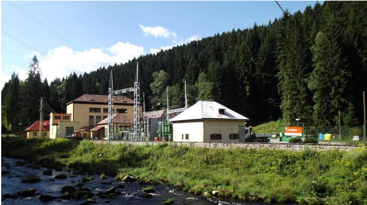
*Figure 20 - Small hydro Vydra 6.4 MW*
