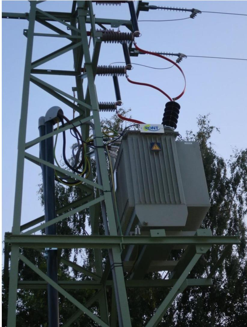
*Figure 50 - Voltage regulated distribution transformer 35/0.4 kV with OLTC installed in Luzany area*
