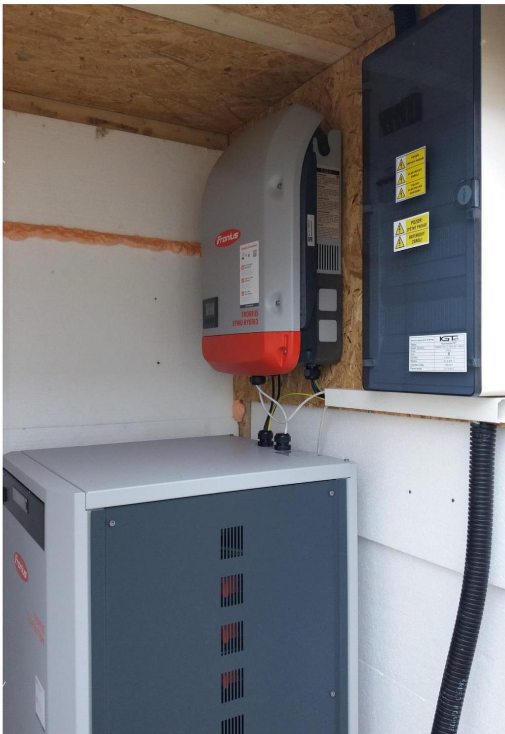
Figure 49 - Fronius smart energy storage system (PV inverter, battery) installed in Luzany area
