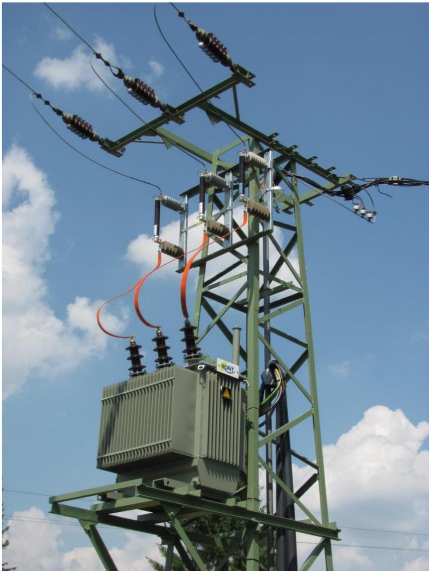
*Figure 15 - Voltage regulated distribution transformer 22/0.4 kV with OLTC installed in Divisov area*
