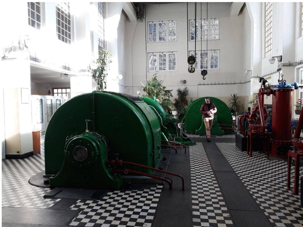
Figure 21 - Small hydro Vydra 6.4 MW - 2 generators which are used for volt/var control (nominal installed power of each generator is 3.2 MW)
