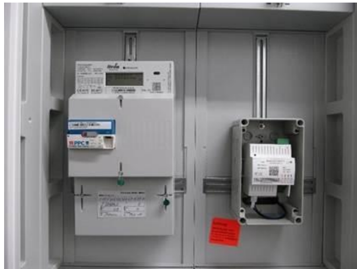
Smart meter with smart meter gateway and the control box to be tested in InterFlex
