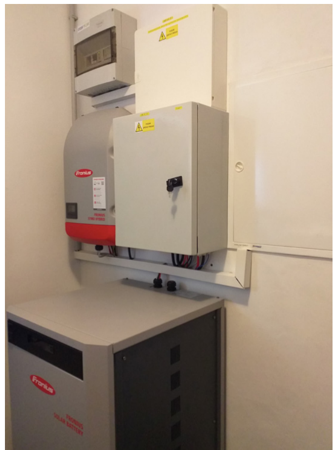
Fronius PV inverter + battery storage system + control box – equipment used for demonstration of smart energy storage concept under WP6
